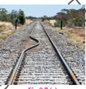
Fig 9.7 (a) Thermal expansion
